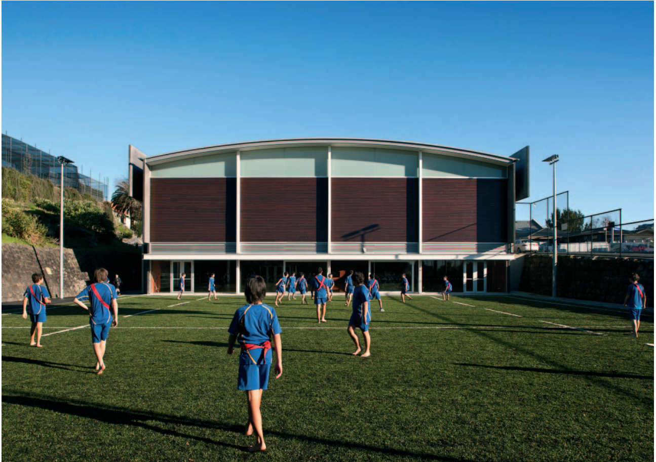
View of Eastern Facade
