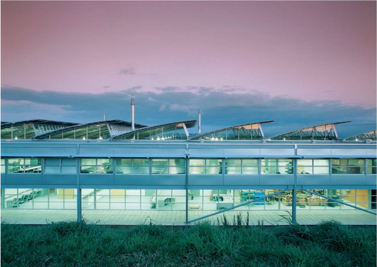
View from the West
