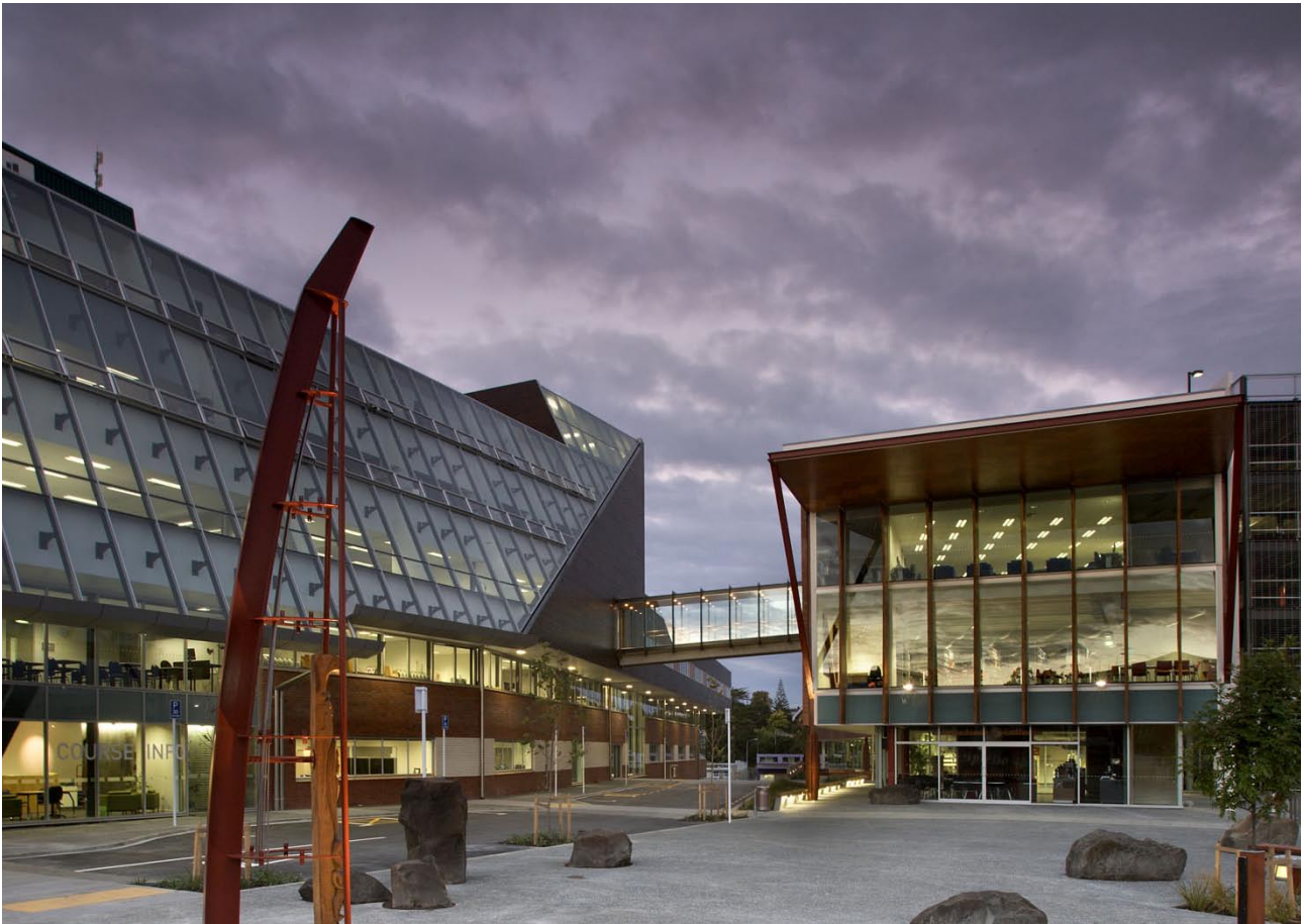
View from Ratanui Street
