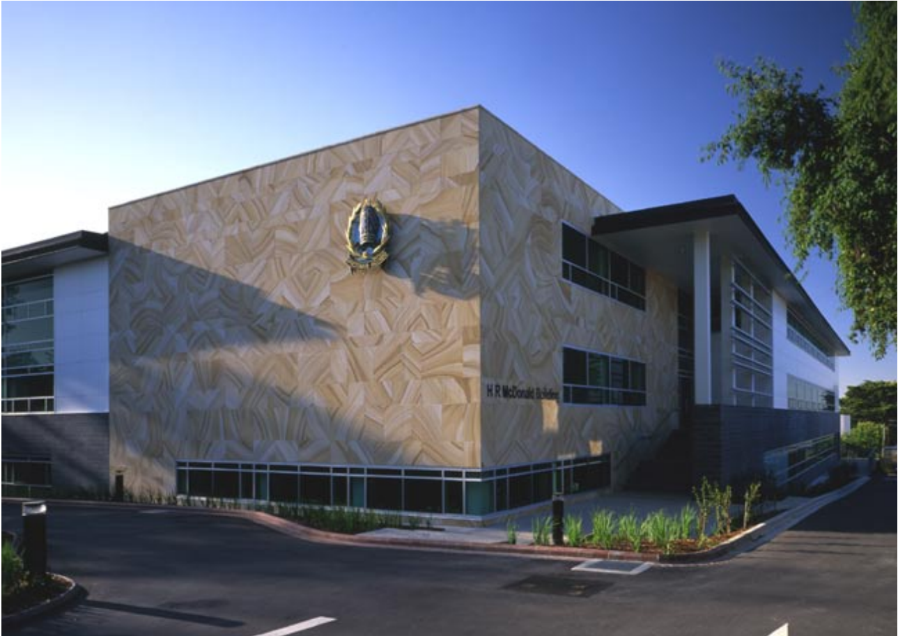
South elevation, gateway entrance
